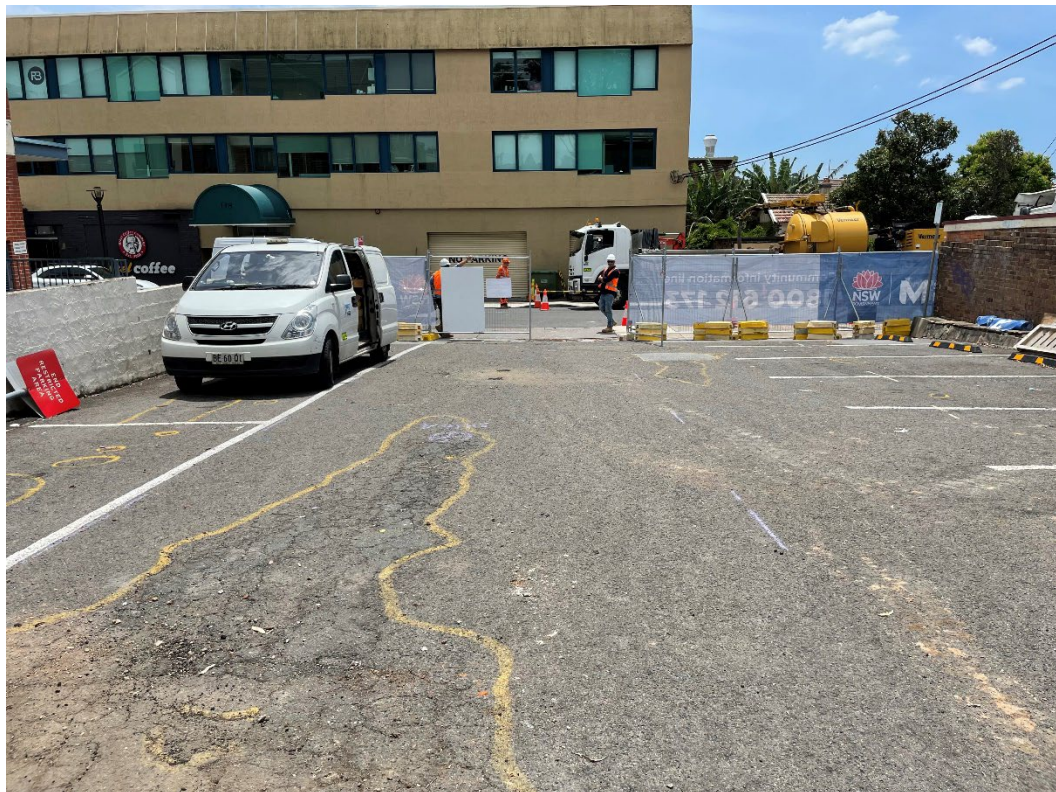
Plate P4: Eastern construction zone car park (facing north)
