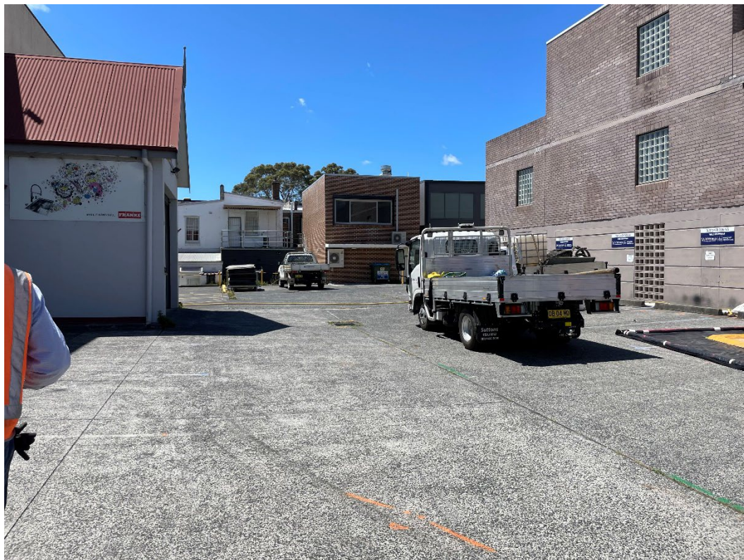
Plate P2: Western construction zone car park (facing east)
