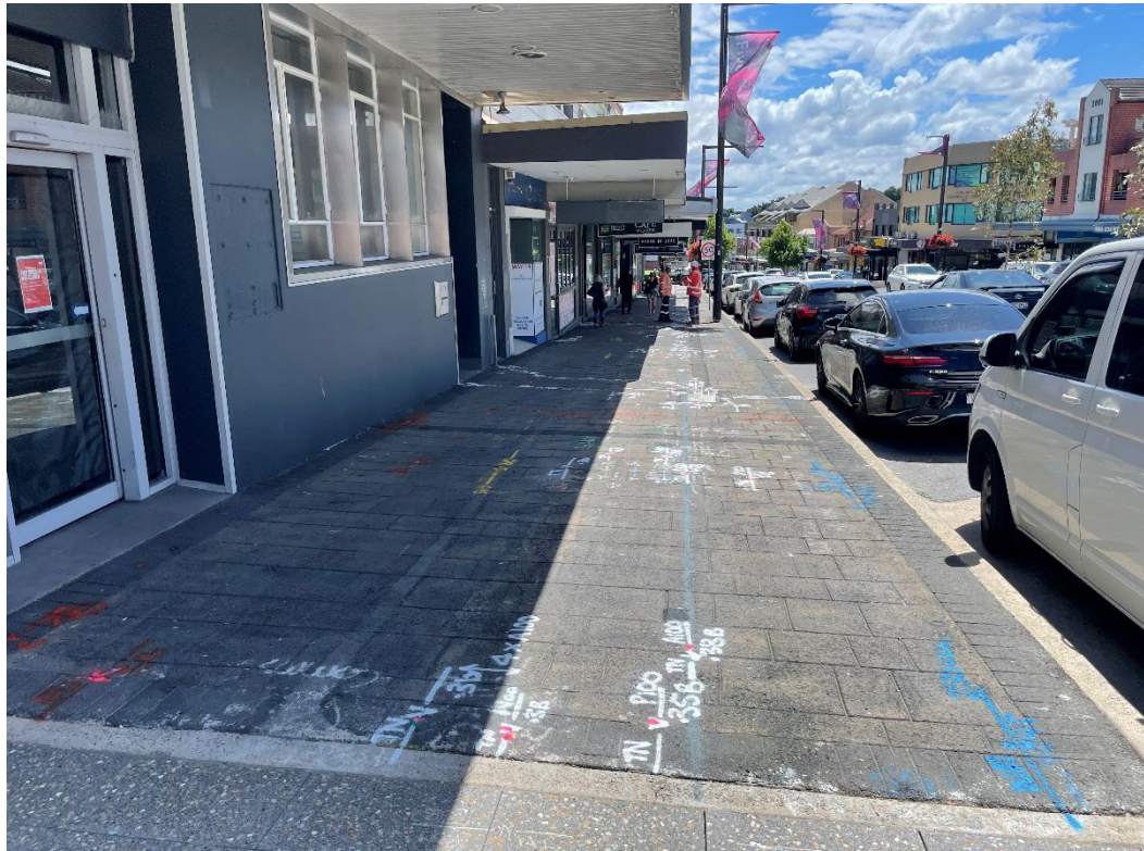
Plate P1: Great North Road, eastern boundary of the western construction zone (facing north)
