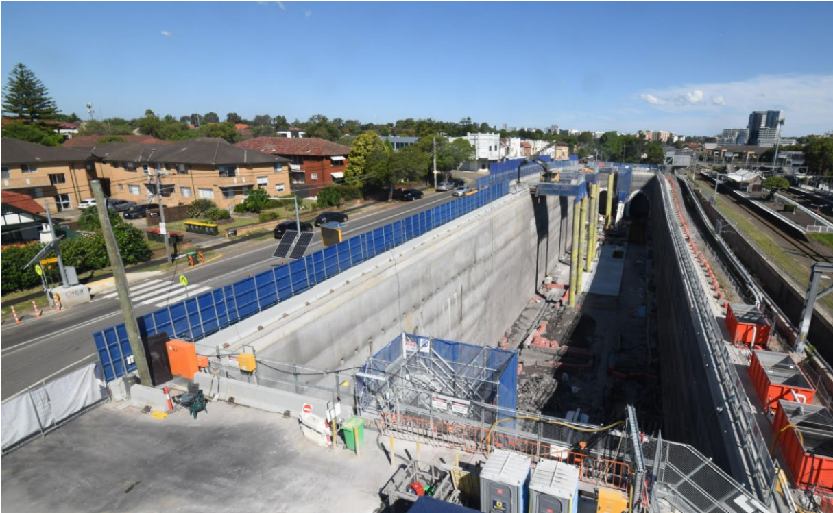
Figure 5-2 North Strathfield Hoarding in situ
