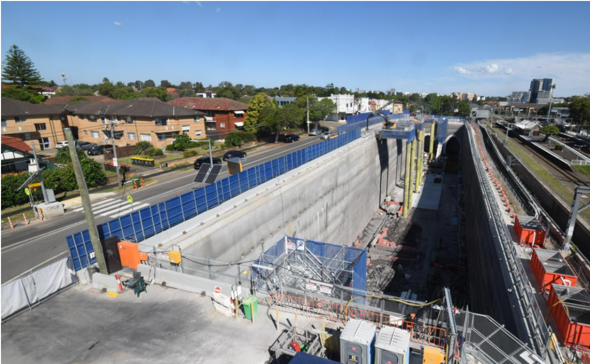
Figure 5-2 North Strathfield Hoarding in situ
