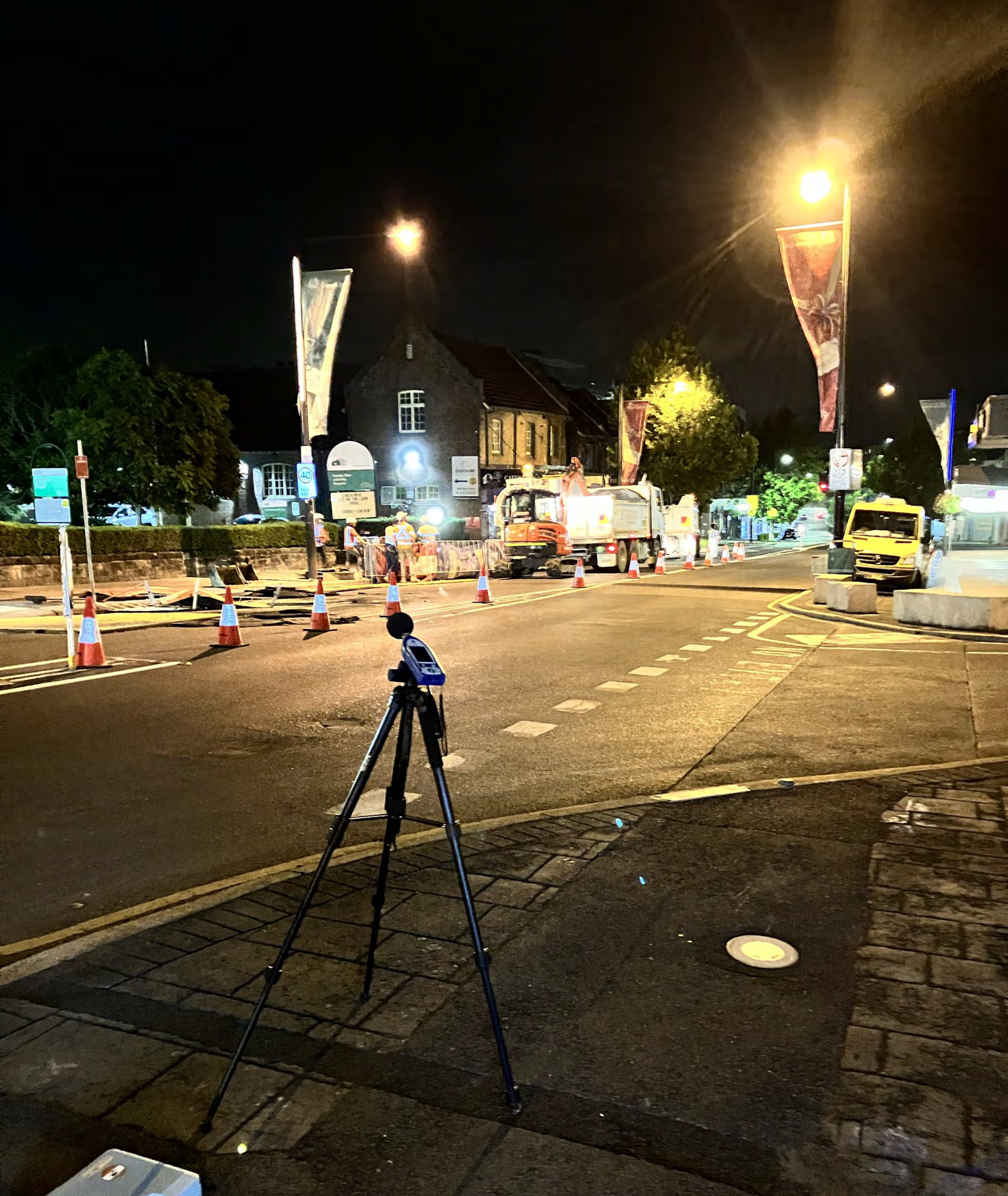
Attended Noise Monitoring Rion-42 - Five Dock
