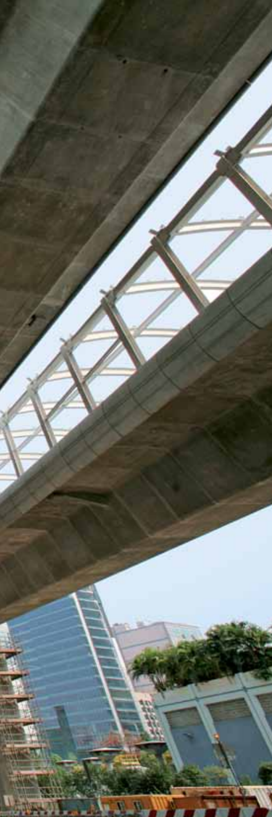
Lai Chi Kok viaduct. Hong Kong, China.
